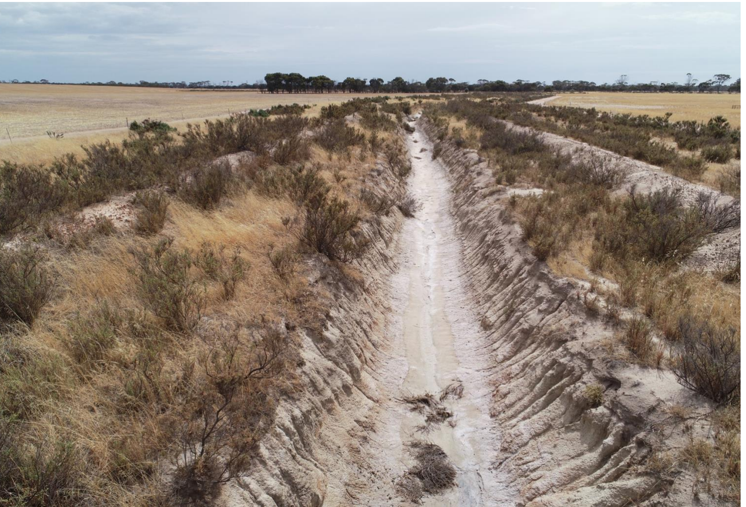
The drainage corridors feature an excavated central channel, batters set back from the channel, with a buffer zone of naturally regenerated vegetation, and then fenced off from the paddock.
